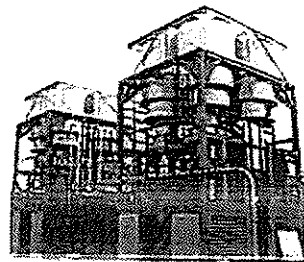
Two CEB 4800* at chemical plant
