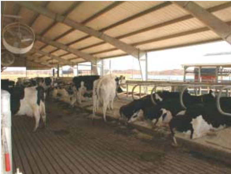
Freestall and Concrete Feed lane
