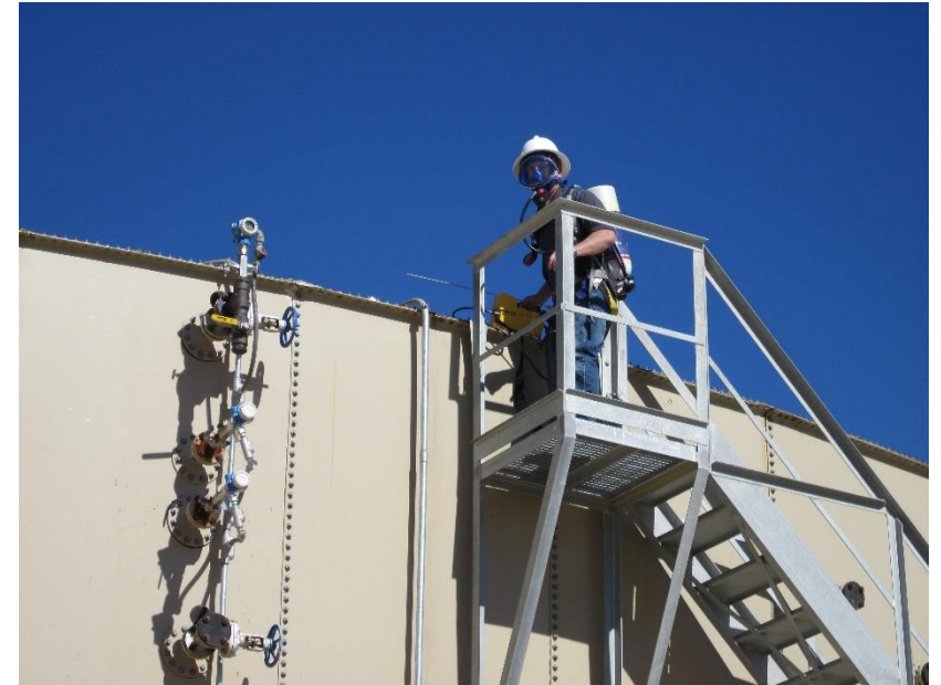
District LDAR tank inspection
